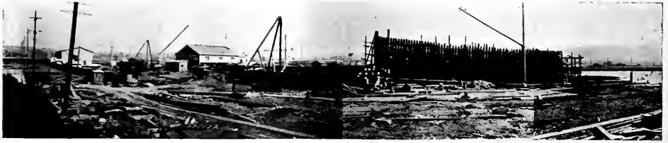
Panorama of the National Shipbuilding Company's plant at Seattle.
